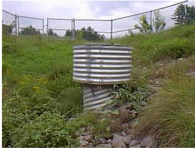
**Figure 4. DOT Retention Basin Outlet (overflow)**
