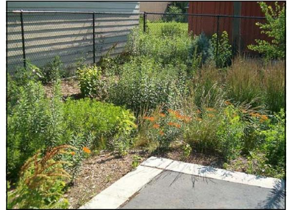
In 2006, the City of Nashua installed a rain garden as part of the site design at the new Public Works facility. Located at the edge of the parking lot, the rain garden catches runoff and reduces pollutants from infiltrating the ground water and Nashua River.
