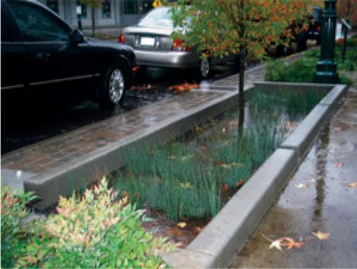
So what are the differences between open and closed systems and how can communities use both of them without impacting the environment or the community? First, let's define the two systems. An open drainage system uses swales and open channels to convey stormwater and is often integrated with Low Impact Development techniques. Closed drainage systems use pipes, culverts and manholes to convey stormwater to detention basins or other centralized infiltration areas.
