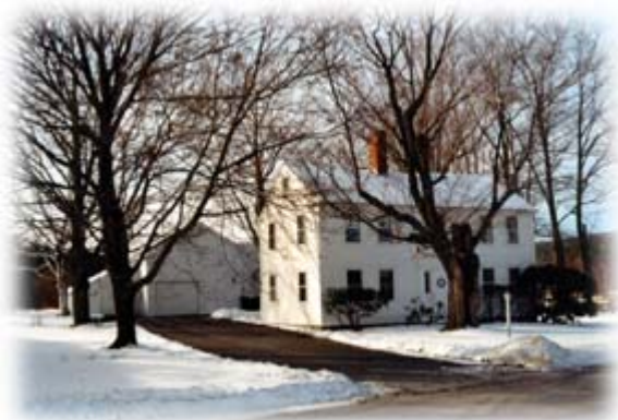
The house on lot 07-29 is of Georgian Style with the garage behind the main building. The main building is one and a half stories and approximately twice as wide as it is deep. Floor area of the main building is approximately 2,000 ft 2 .
