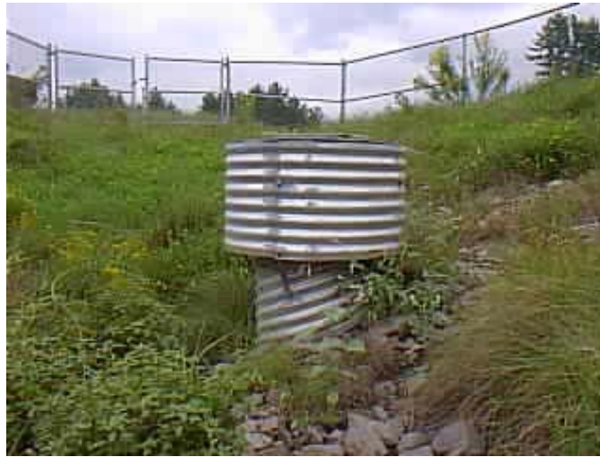
Figure 4. DOT Retention Basin Outlet (overflow)
