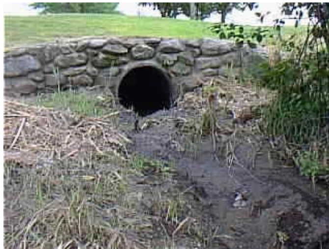
Figure 5. Somerset Plaza Swale Inlet
