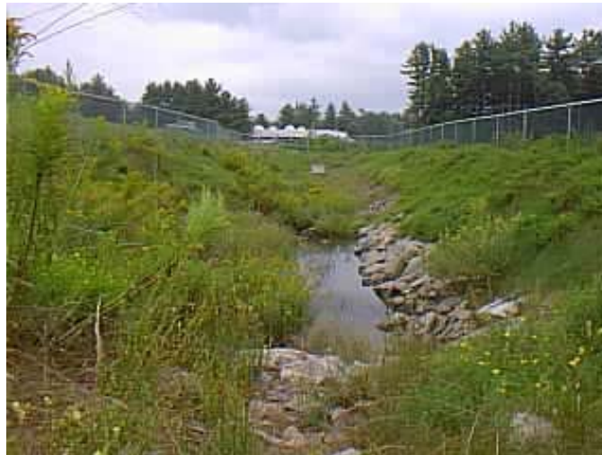
Figure 3. DOT Retention Basin Inlet
