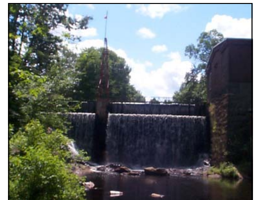
Chamberlain Mills Dam in Greenville NH.
