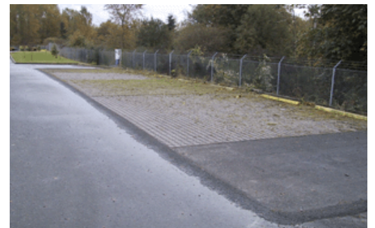
Permeable Parking Lot Demonstration - Open Drainage Seattle, WA
