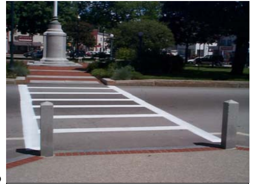
Curb Extensions, like this one in Milford, reduce crossing distances for pedestrians. Photo: NRPC
